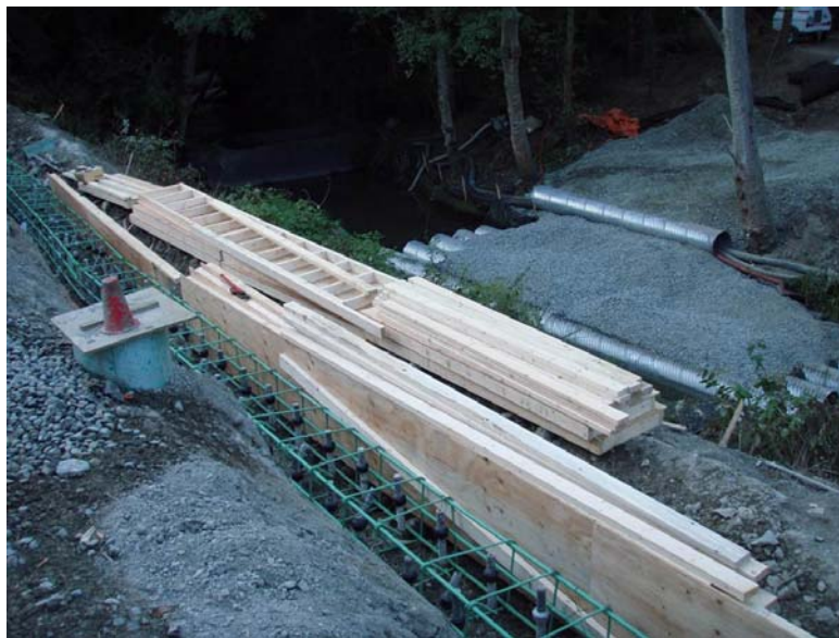
Figure 10. The completed micropiles, cap steel and cap forms during assembly.
