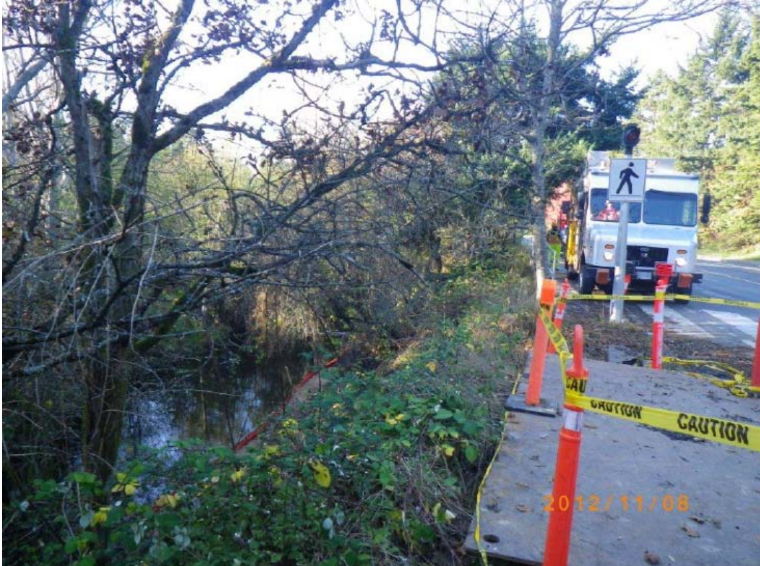
Figure 2. Site photo showing the easement and existing Colquitz Creek embankment.
