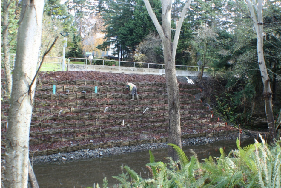
Figure 12. Completing the living earth wall.
