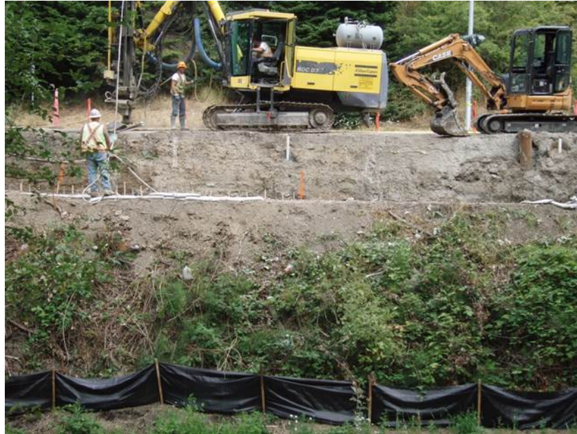
Figure 9. Drilling the micropiles at the crest of the partially excavated slope.
